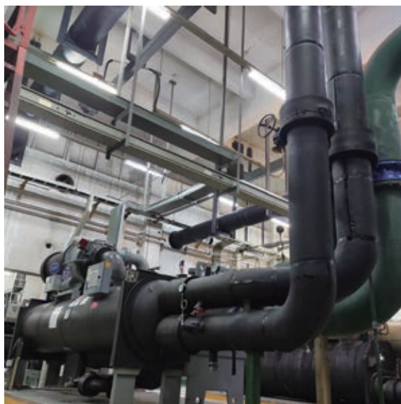
Refrigeration station pipeline renovation
